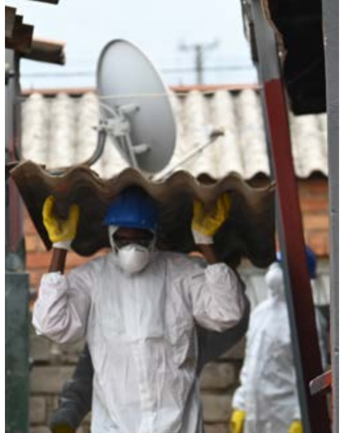
Worker in full protective gear carefully removing an old asbestos roofing panel.
