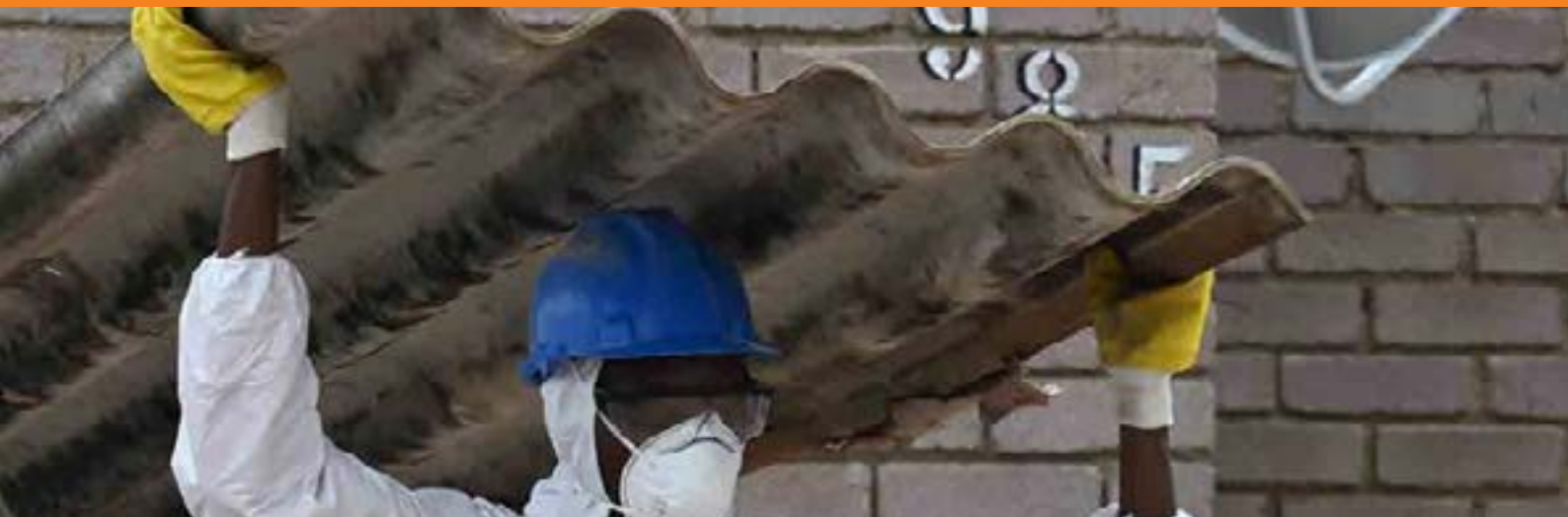
Worker in full protective gear carefully removing an old asbestos roofing panel.
